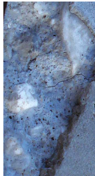
b) Microcrack in a pillar of the Holocaust Memorial, Berlin
