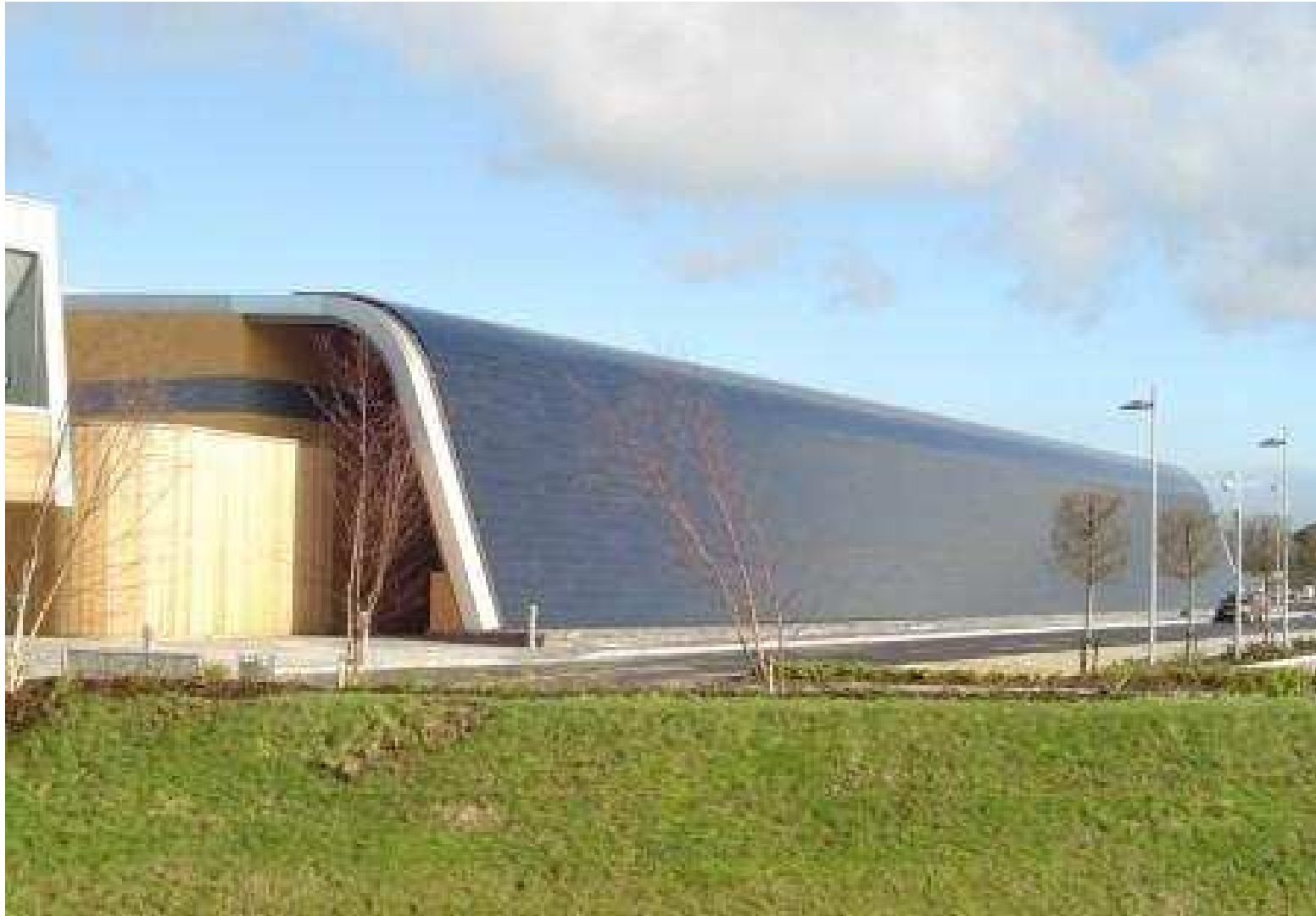
Optic Center Wales, CIS-Module, 85 kW p , 2004
